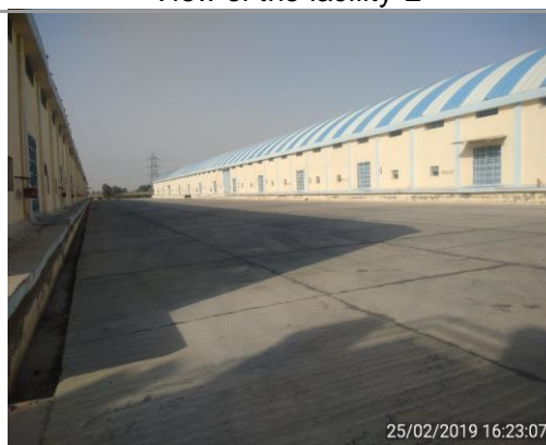
View of the facility-4
