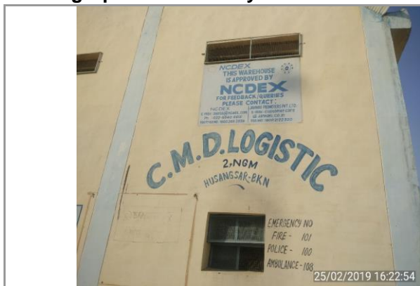
View of the facility-1
